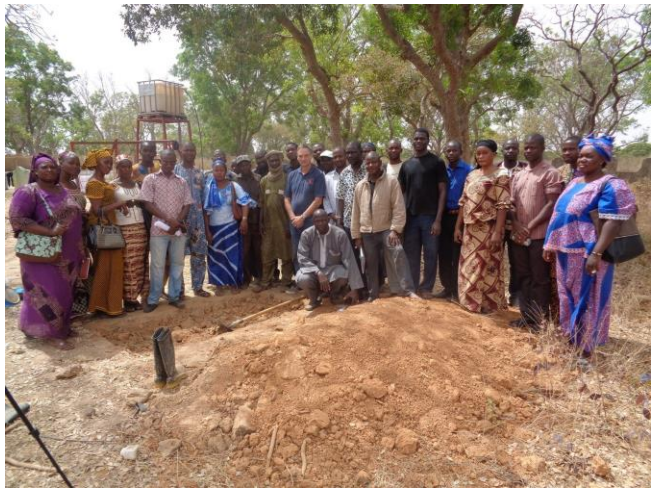
Finished, covered silage pit.
